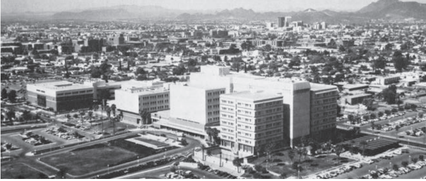
The University of Arizona Medical Center, 1983.
